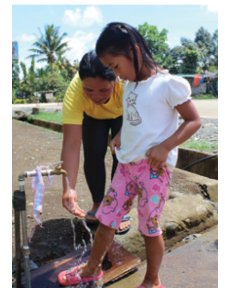
Water system installed in a locality
