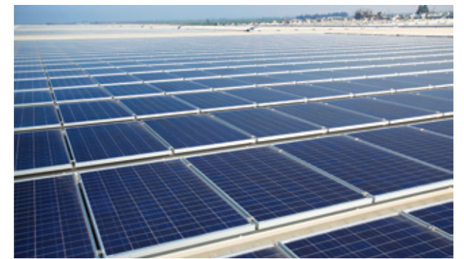
Solar panels in Hanford facility in California, USA
