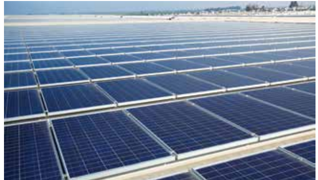
Solar panels in Hanford facility in California, USA
