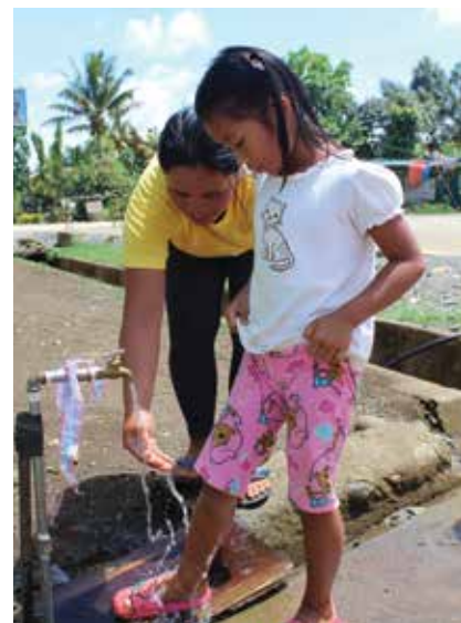
Water system installed in a locality
